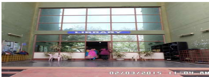
Photo shows entrance of 3 storey independent Library building:
